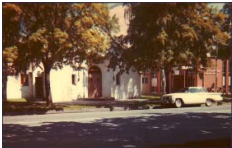
First Lutheran - August 1962 - before remodeling of the church.
