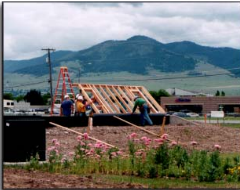
Raising of the first wall of our new church.
