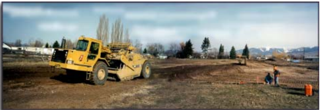
March 17, 1999 - beginning of ground work at our new church site.
