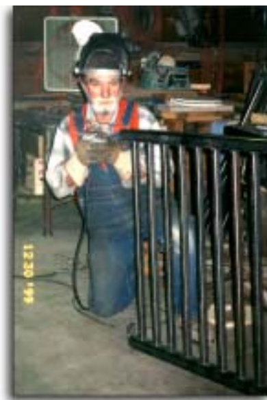
Norm Balko in his garage welding the rail for the choir loft area.
